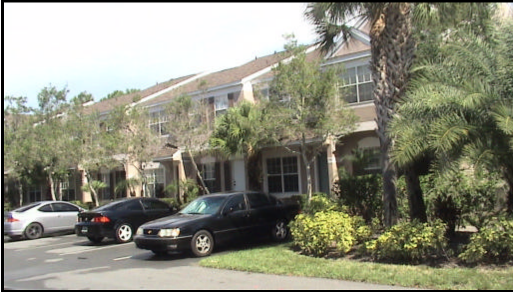
The front of Building I Phase 1 a ten unit building
