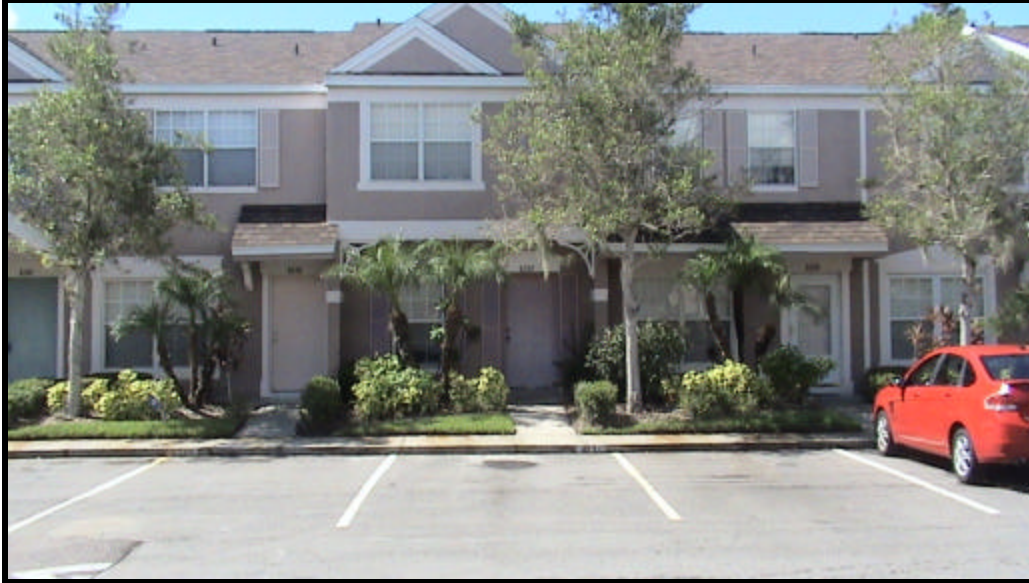
The front of Building L Phase 2
