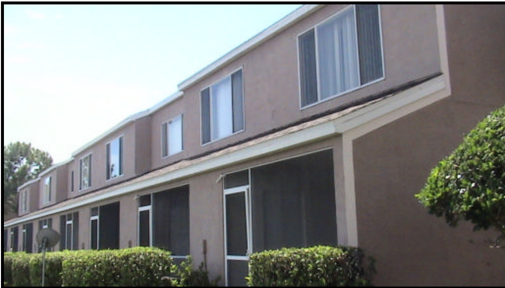
The rear of Building H Phase 1
