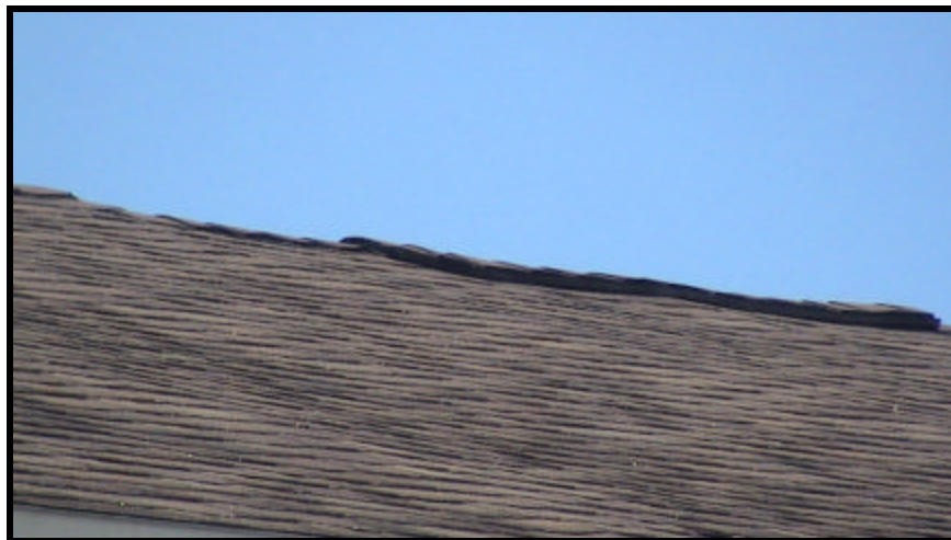
The roof of one of the buildings
