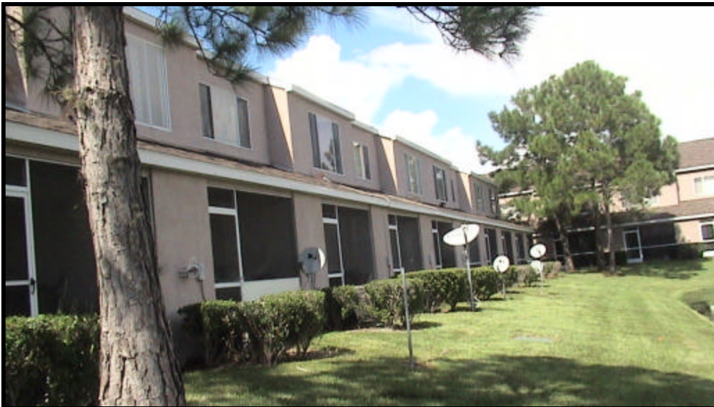
The rear of Building I Phase 1
