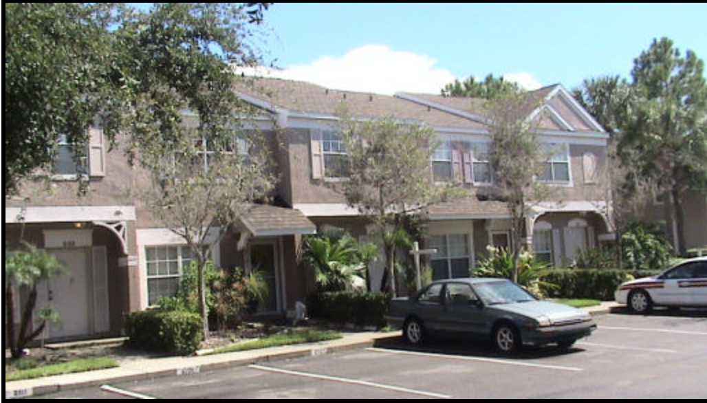
The front of Building H Phase 1 a ten unit building
