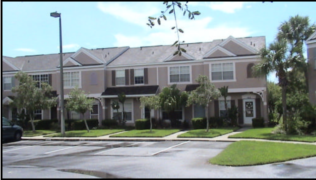
The front of Building C Phase 1
