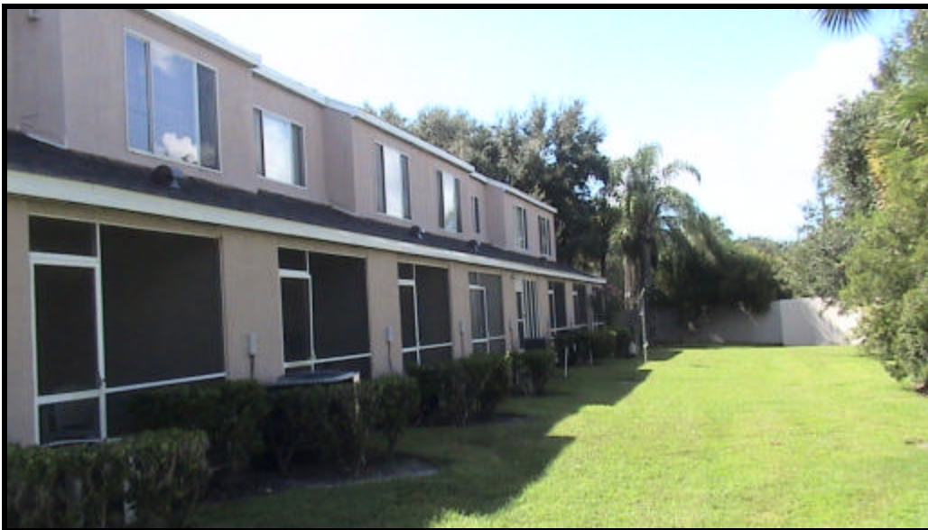
The rear of Building S Phase 2
