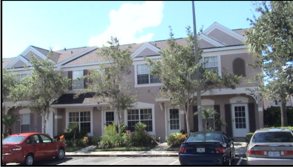
The front of Building M Phase 2
