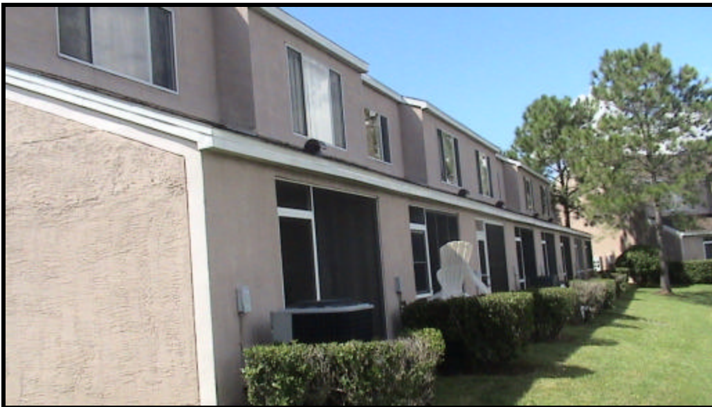
The rear of Building G Phase 1
