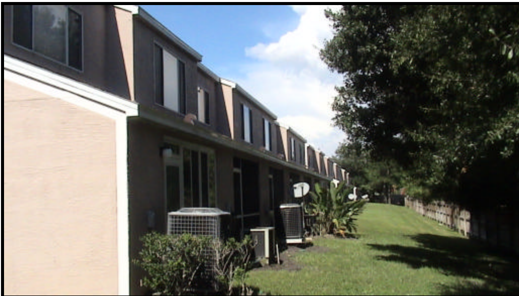
The rear of Building O Phase 2
