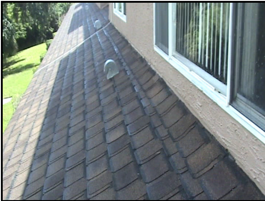
The roof of one of the buildings
