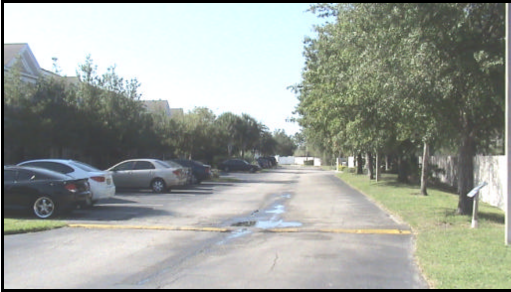
The ingress / egress easement and Bayside Key Drive
