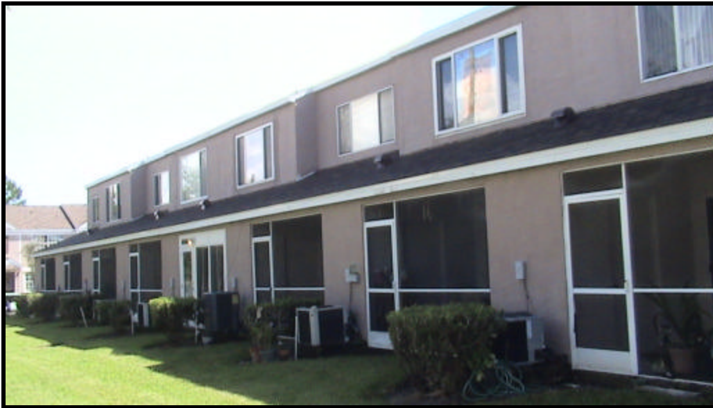
The rear of Building R Phase 2
