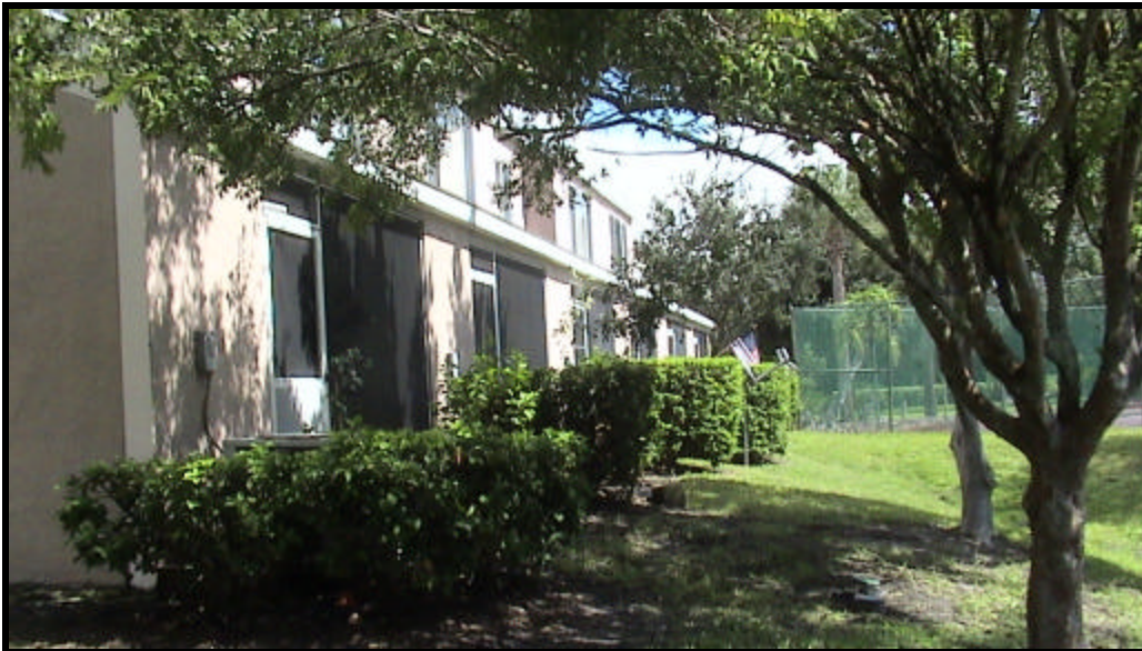
The rear of Building C Phase 1
