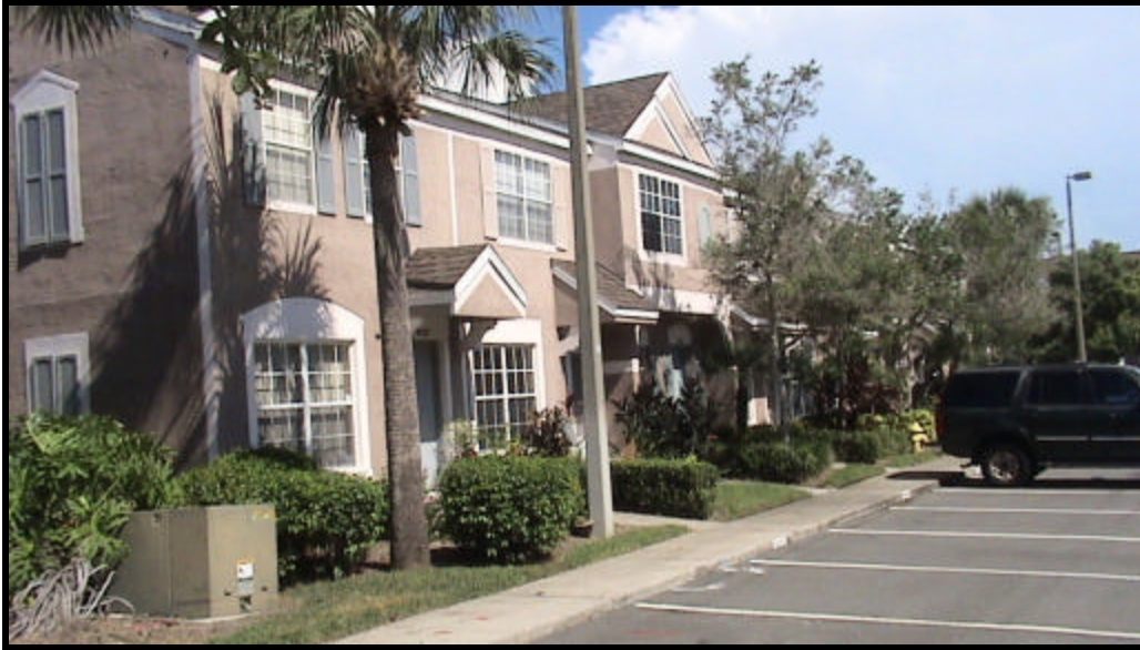
The front of Building R Phase 2
