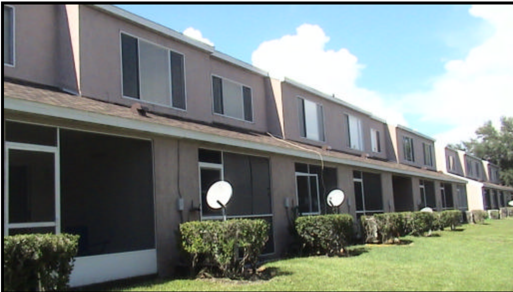
The rear of Building P Phase 2
