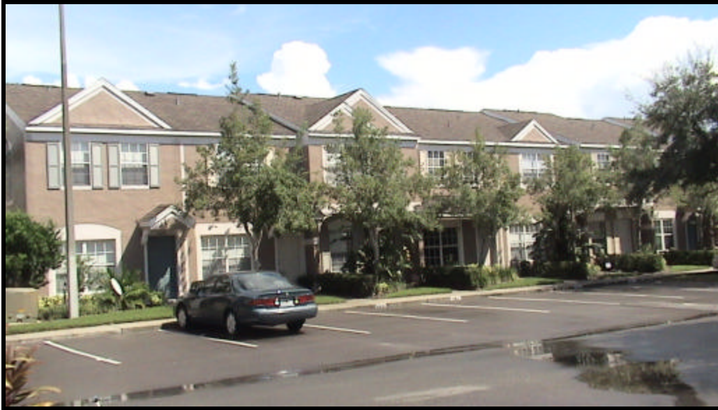
The front of Building D Phase 1
