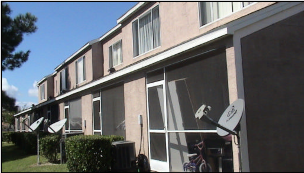
The rear of Building J Phase 2
