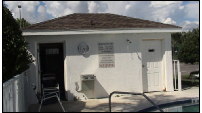
The Pool House containing full men and women's restrooms with showers
