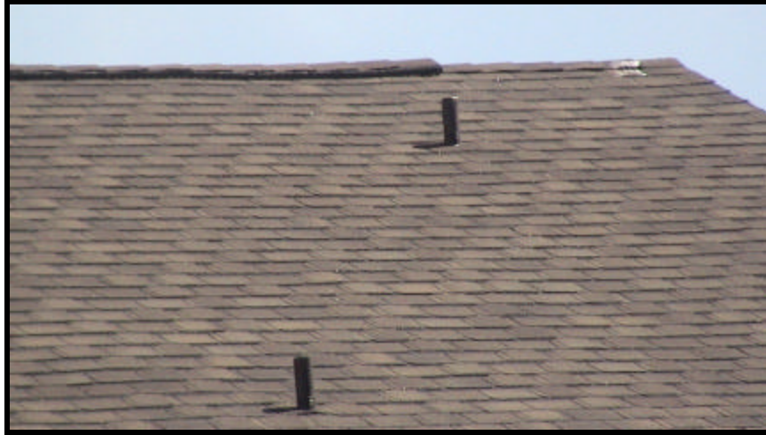
The roof of one of the buildings
