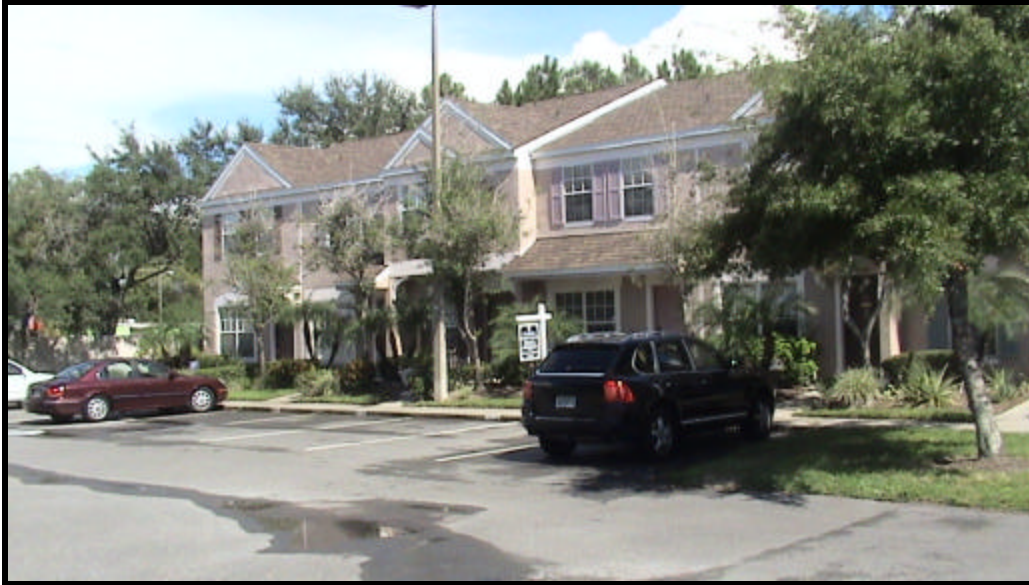
The front of Building Q Phase 2
