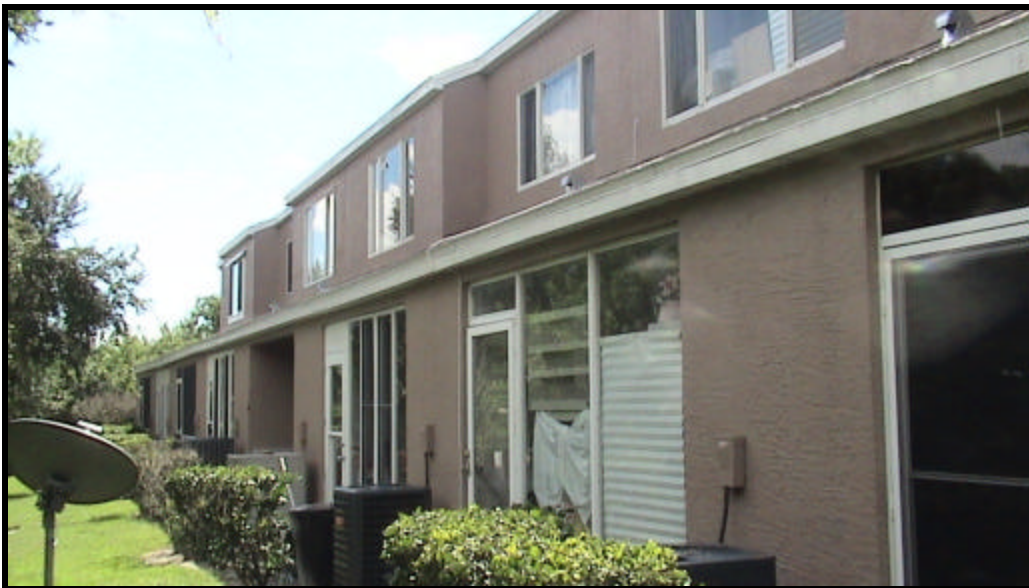
The rear of Building D Phase 1
