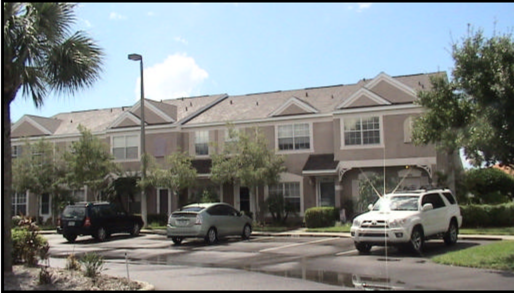
The front of Building B Phase 1
