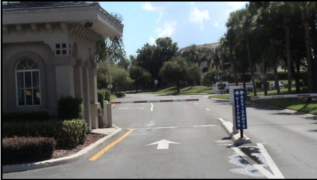
The security gate of the subject property's neighborhood
