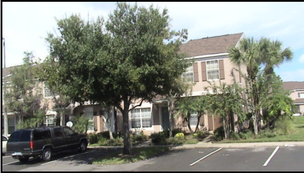
The front of Building G Phase 1
