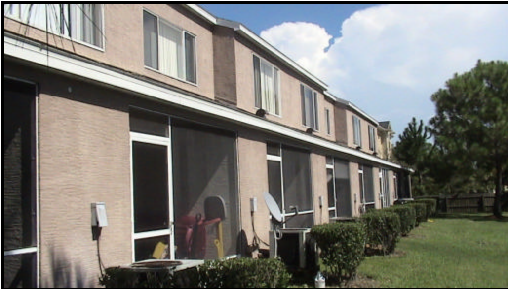
The rear of Building N Phase 2
