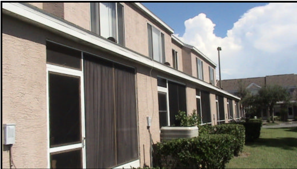
The rear of Building J Phase 2
